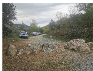
Manrell pass road
